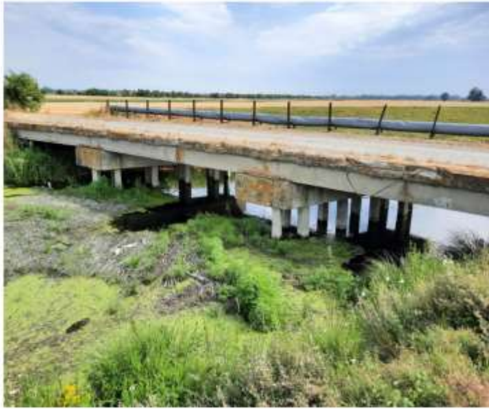
Photo taken July 2023: bridge prone to vegetative debris
