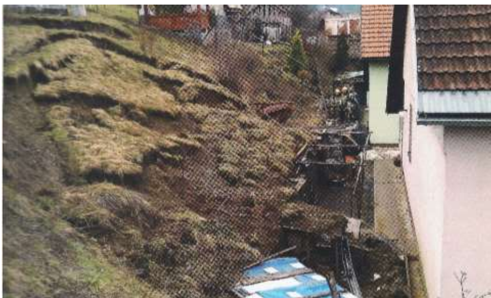
Fig. 4: Landslide threatening a family house [7].
