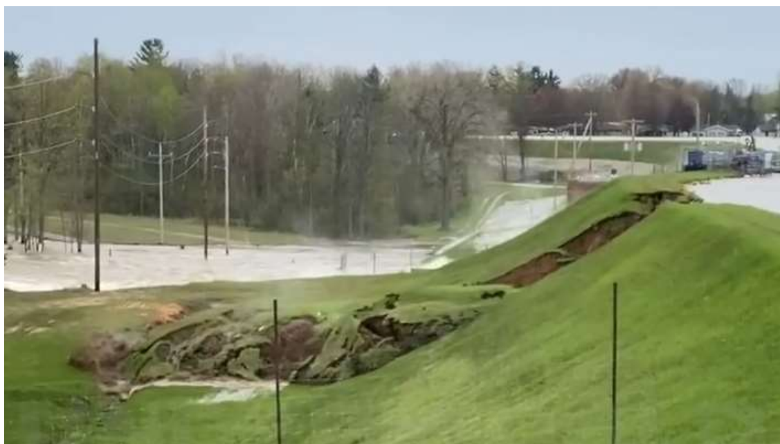
Fig. 2 The failure of the Edenville Dam, USA [3].
