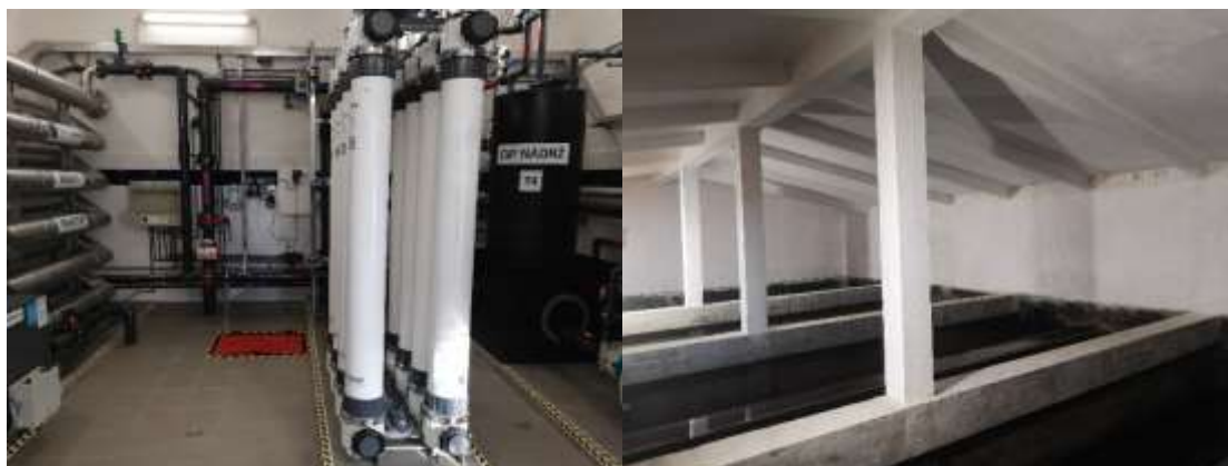
Figure 1 Štrbské Pleso WTP – view into the WTP with ultrafiltration modules (left), Štôla WTP – hall with slow sand filters (right)
