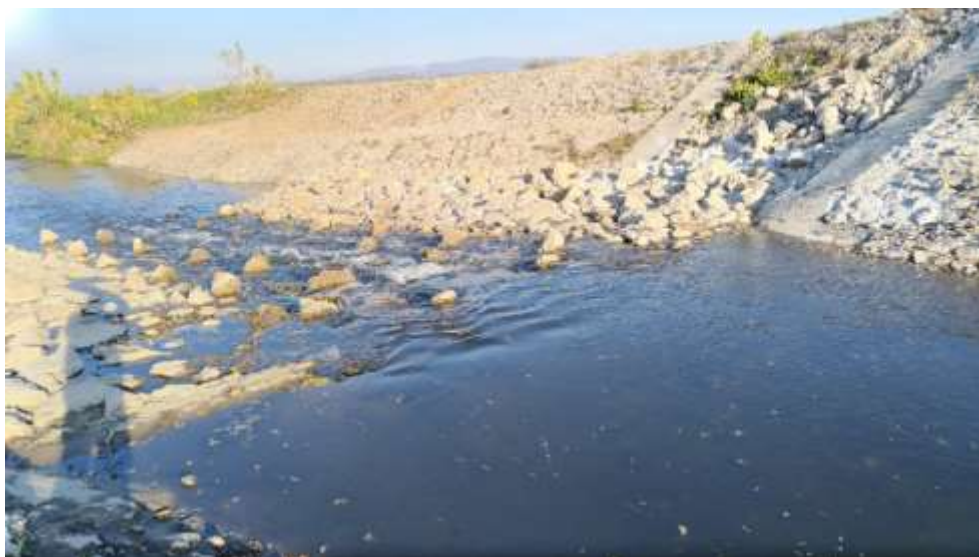
Figure 13 Built rock ramp fish pass [8]
