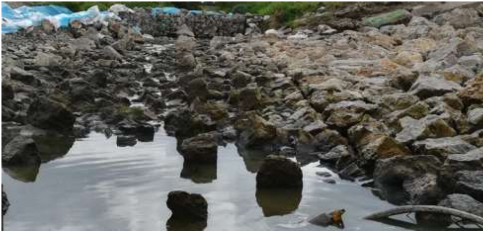
Figure 14 Boulders on the river bed bottom of the fish pass
