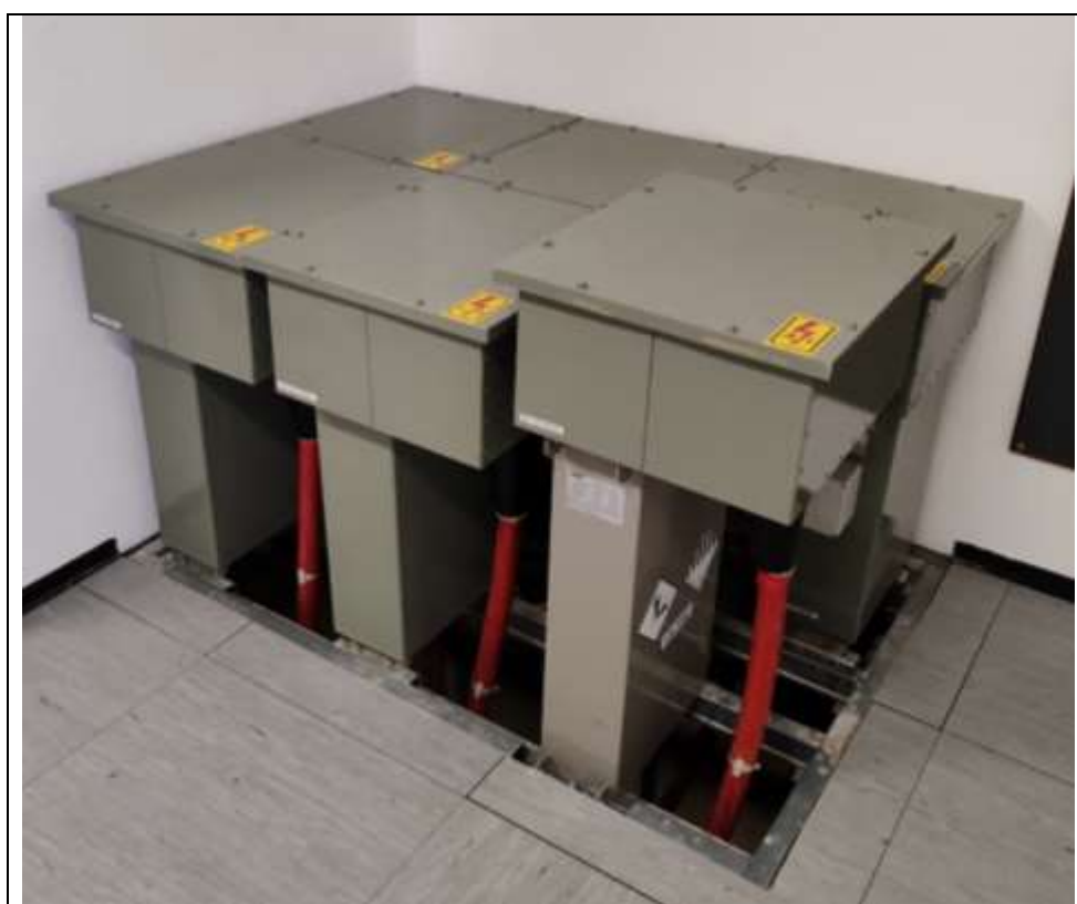
Figure 4. Capacitors units on DWTF Butoniga.
