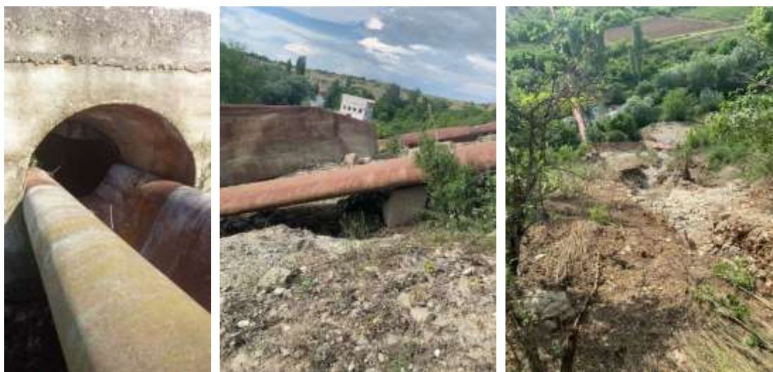
Figure 1. Pipeline break under pressure - siphon caption heading
