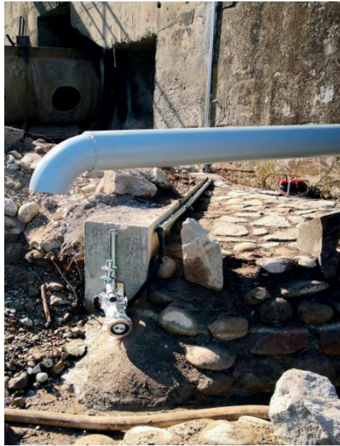
Figure 4. Cameras at the inflow and outflow (construction state)
