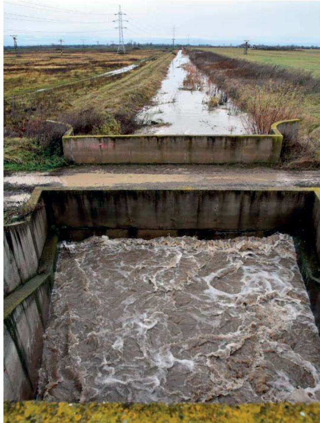
Figure 3. Culvert on the Trnávka River, rkm 9,380 (photo Mydla)
