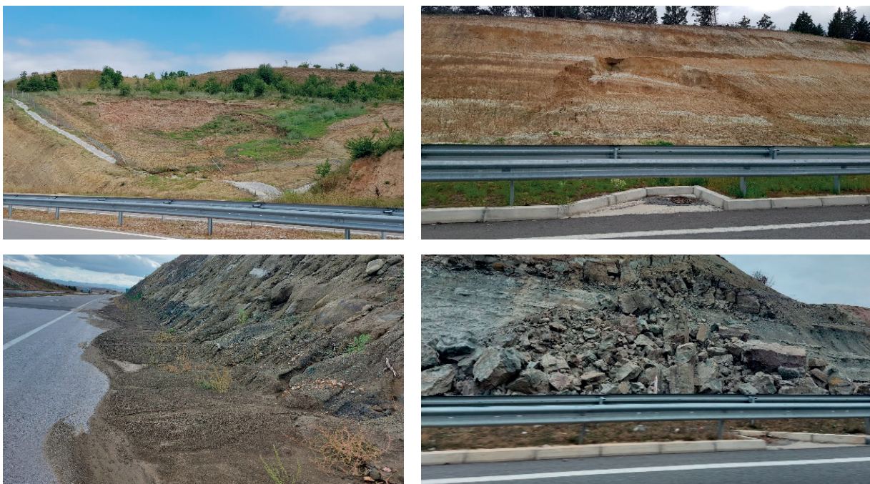
Figure 1. Slope stability problems on Miladinovci – Shtip highway
