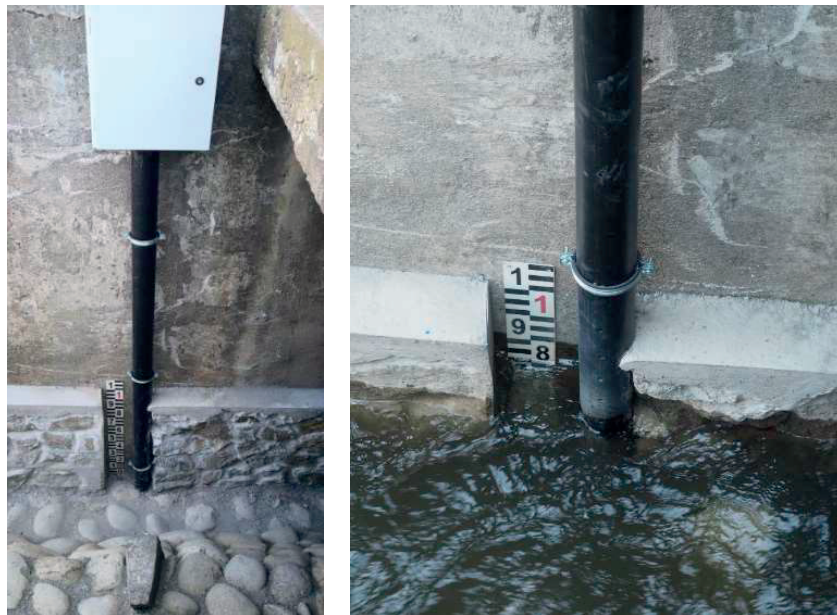
Figure 3. Probe for continuous water level measurement (staff gauge, data logger)
