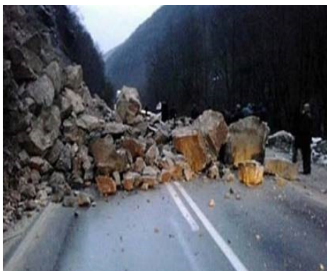
Rockfall on the road Kochani – Shtip in 2013
