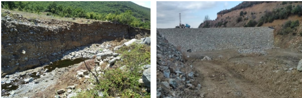
Figure 6. Reconstruction of Drenska Dam.
