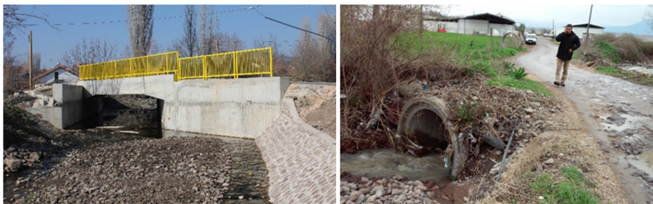
Figure 3. Recovery of culvert in the municipality of Cesinovo-Oblesevo (before and after)
