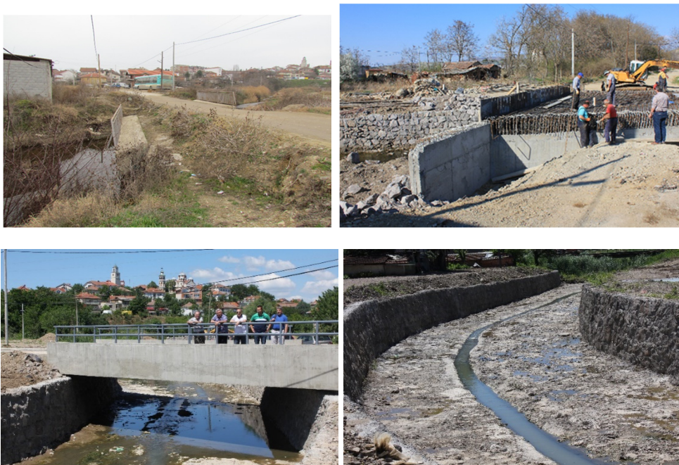
Figure 5. Bridge in the municipality of Sv. Nikole and new river regulation to enhance discharge capacity
