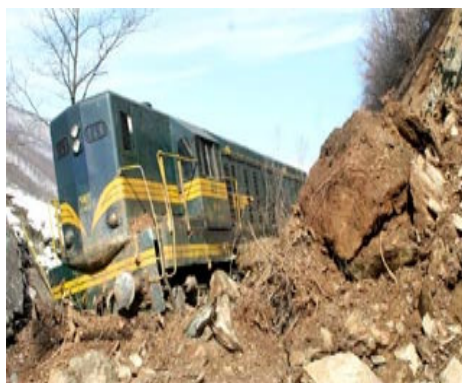
Rockfall on the railway Gostivar – Kichevo in 2010
