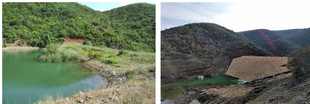
Figure 4. Reconstruction of Lipa Dam
