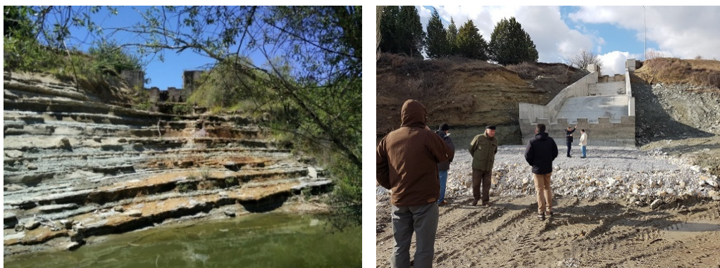
Figure 3. Reconstruction of spillway and stilling pool of Mavrovica Dam
