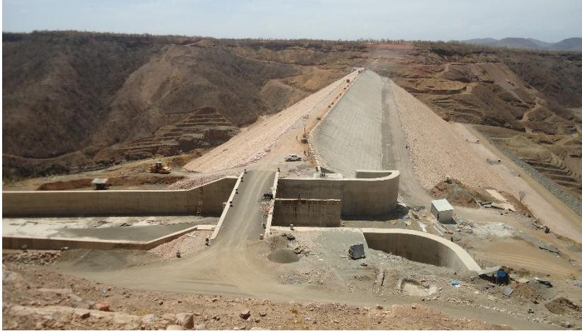
Figure 9. Works under completion at Zarema May Day dam
