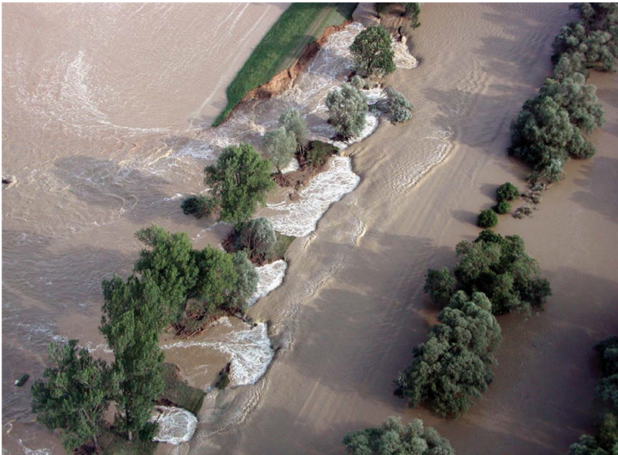
Figure 2. Protection dyke breakage on the Ondava River (July, 2004)
