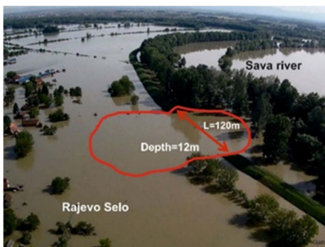
Figure 10 Breach of a Sava River dyke with an extensive scour on the landside (120 x 300 x 12m) due to internal erosion of the ground below the dyke in 2014 [20].
