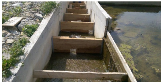
Figure 1. Conversion of baffle fishway into pool fishway on SHPP Ilovac
