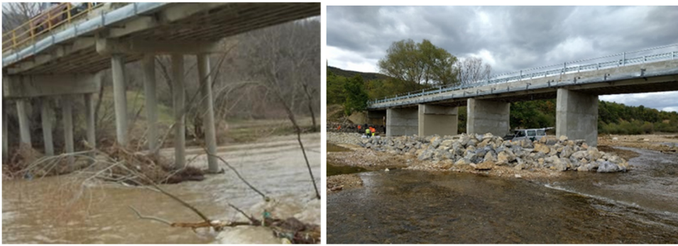
Figure 3. Recovery of bridge in the municipality of Delcevo
