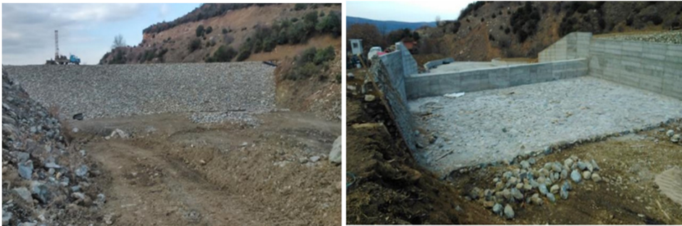
Figure 8. New dam body and a spillway structure on Drenska Reka Dam
