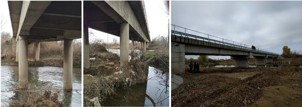
Figure 4. Recovery of bridge in the municipality of Zrnovci
