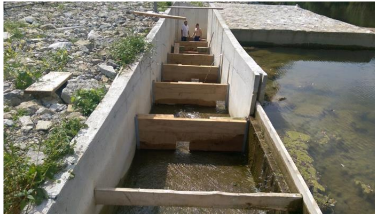
Figure 2 Pool fishway at SHPP Ilovac under construction
