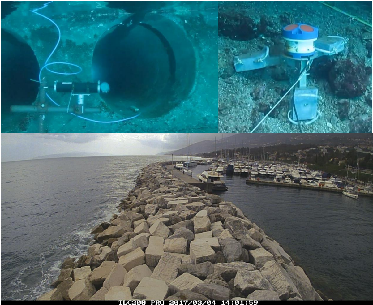
Figure 8. PCM and CTD probe at the culvert; ADCP2 at the leeward side of the culvert; snapshot of the time lapse camera located at the head of the breakwater
