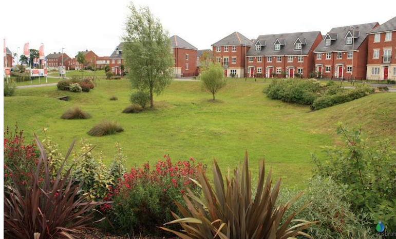
Figure 3. Example of stormwater detention pond (basin) [10]
