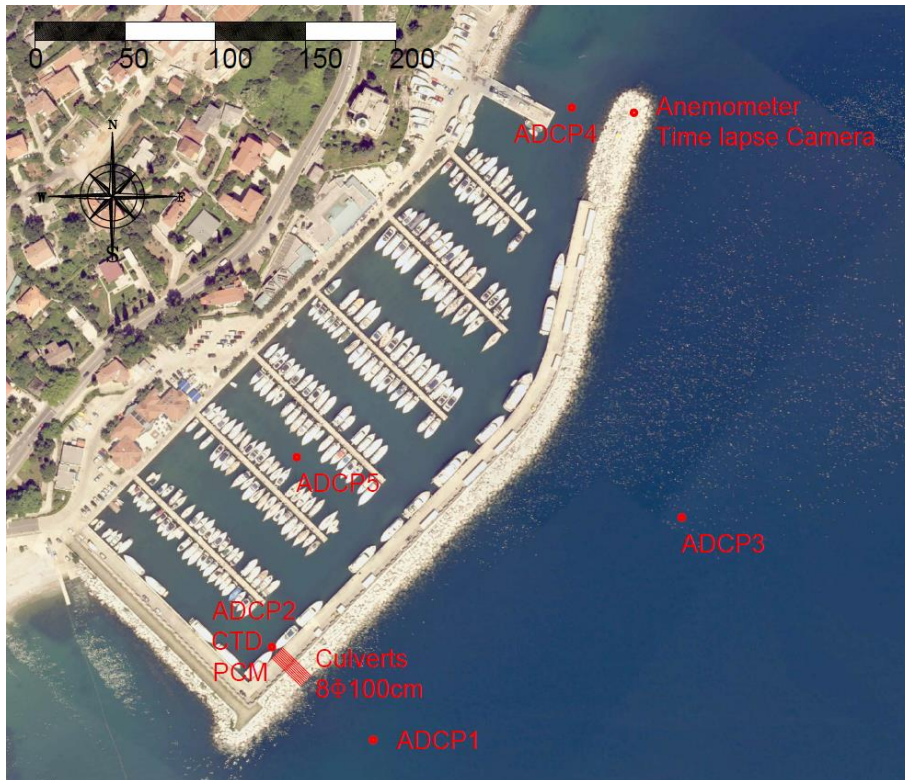
Figure 5. Layout of measuring devices in small marina Opatija; ADCP- sea current profiler, CTD- salinity and temperature; PCM- velocity and discharge in the flushing culvert; Anemometer – wind magnitude and direction
