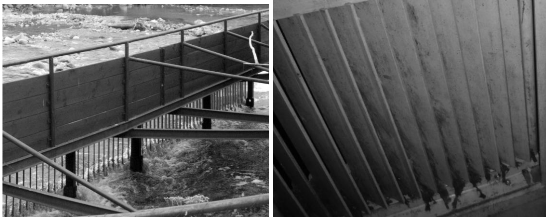
Figure 1. Prototypes of inclined bar racks in Slovakia (Roveň, Pezinok)
