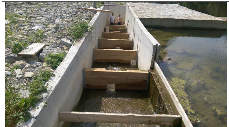
Figure 1. Pool fishway at SHPP Ilovac under construction
