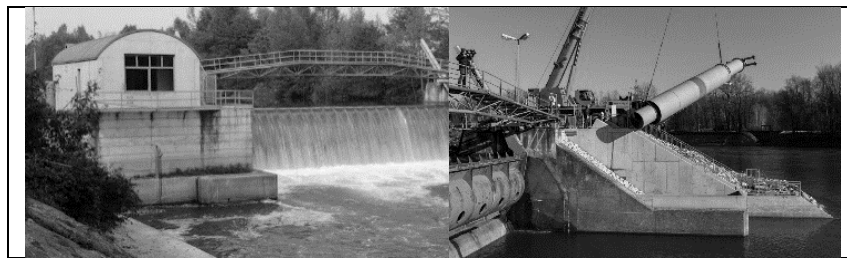
Figure 1. View of the Retznei barrage with the old hydro power plant (on the left) and the new installation of the hydro power plant with the tube-type double rotating screw on the left bank side (on the right).
