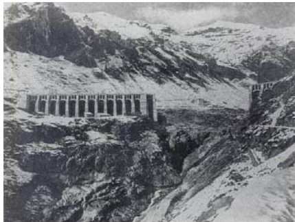
Fig. 2 Gleno dam(1923), collapse of dam block [Herzog, 1999]
