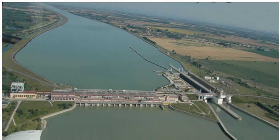
Fig. 2 Hydraulic Structure Gabčíkovo
