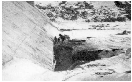
Fig. 4 Ashley Brook Dam (1909), foundation failure [Vogel, 2013]
