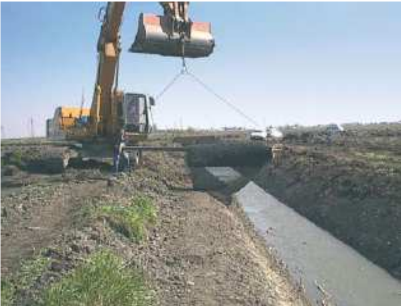
Fig. 5 Installation of beaver netting along Canale Zabarelle
