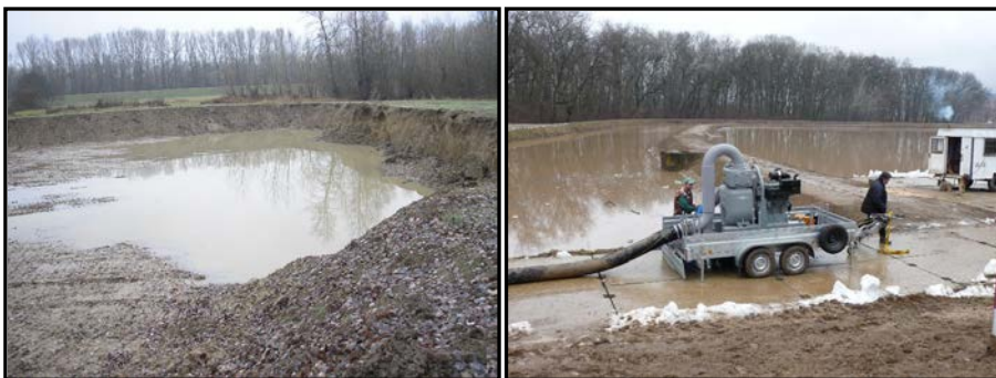
a) excavation of material from pit
