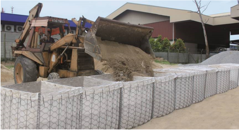
Fig. 9 Filling of FLEXMAC unit [photo Maccaferri Central Europe]
