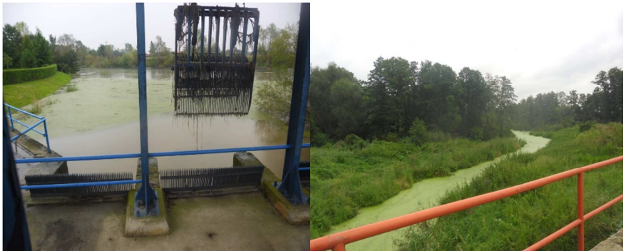
Fig. 3. Eutrophication and sedimentation caused by the “Syphon” (left) and Eutrophication impact in Stream Želin (right)
