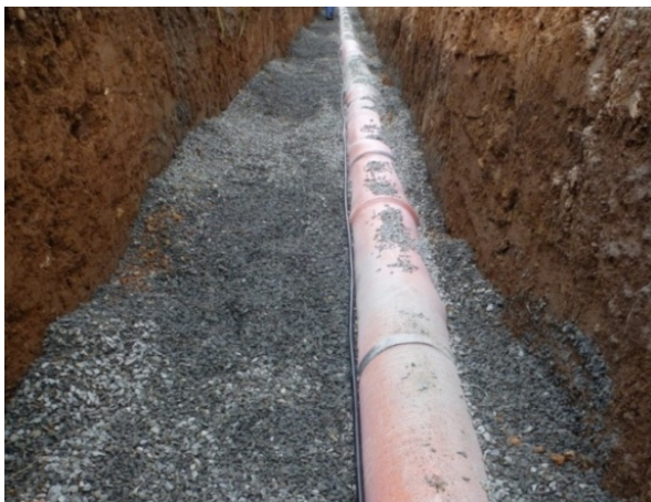
Fig. 2 – Fibre optic cable installation along a new toe drain
