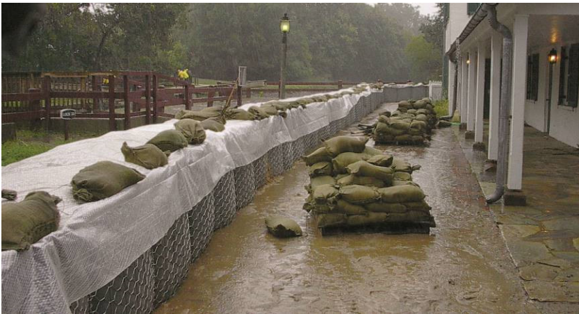
Fig. 10 Application of FLEXMAC system [photo Maccaferri Central Europe]
