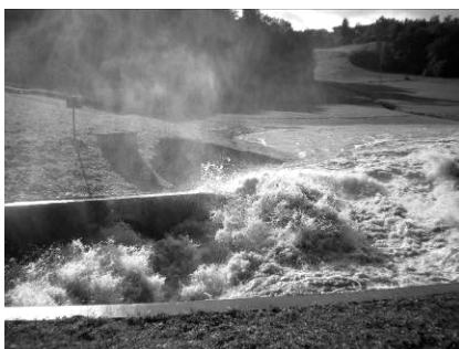
Fig. 4 Outflow from the bottom outlet during the floods in September 2010
