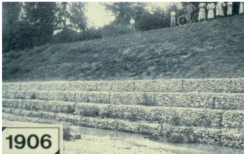
Fig. 2 Historical longitudinal gabion wall at river, year 1906 [photo Maccaferri Central Europe]
