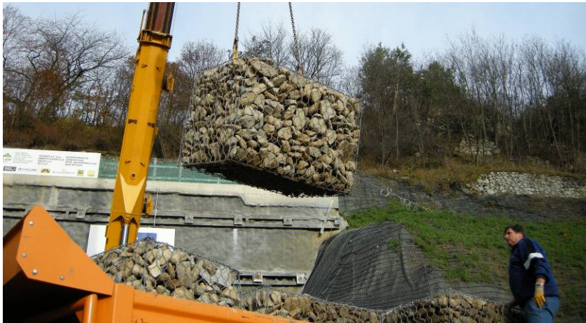
Fig. 8 Installation of CUBIROCK gabion [photo Maccaferri Central Europe]
