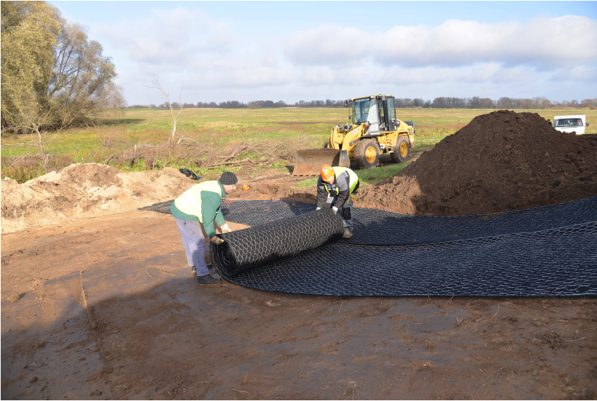
Fig. 4 Installation of beaver netting
