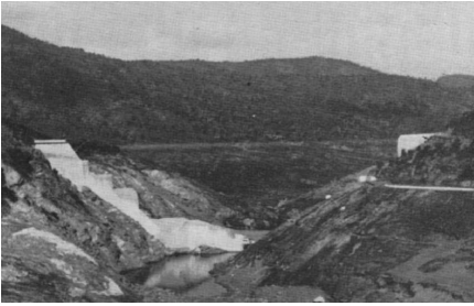
Fig. 3 Malpasset Dam(1959), foundation failure [Duffaut, 2013]
