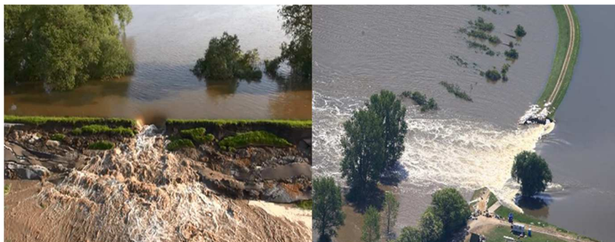
Fig. 2 Levee breaches at Breitenhagen (Saale River) and Fischbeck (Elbe River)
