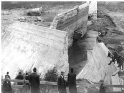
Fig. 1 Bayless Dam (Austin dam) (1911), block sliding [Vogel, 2014]
