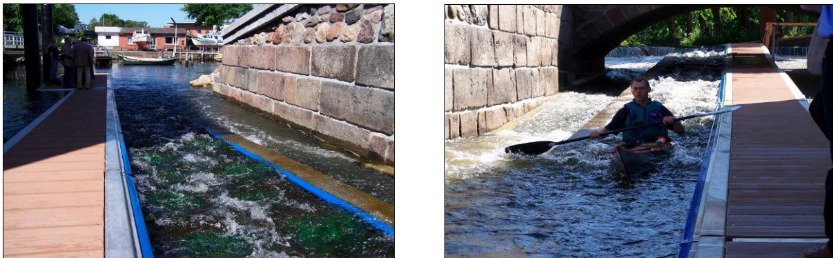
Fig. 9 Bristled fish pass combined with canoe chute [14]
