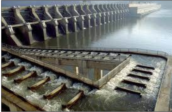
Fig. 6 Slot fish pass [10]
