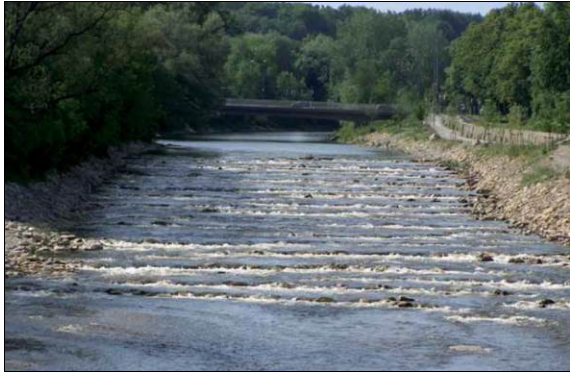
Fig.1 Boulder chute [7]
