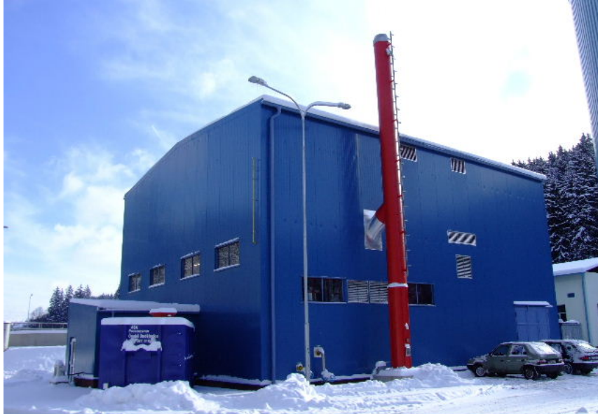
Fig. 1 Incineration station based on sludge burning on fluid layer
