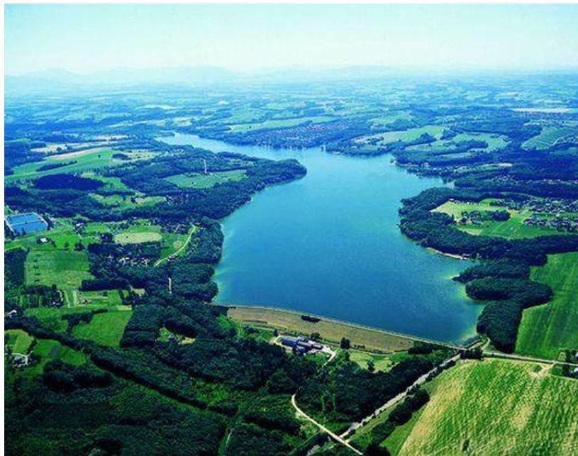
Fig. 2 View of the Terlicko dam (source: www.vzsterlicko.cz )
