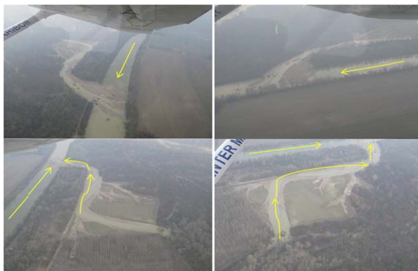
Fig. 8 Downstream levee breach of HPP Formin outlet canal (photo taken 9/Nov/2012) [1]
