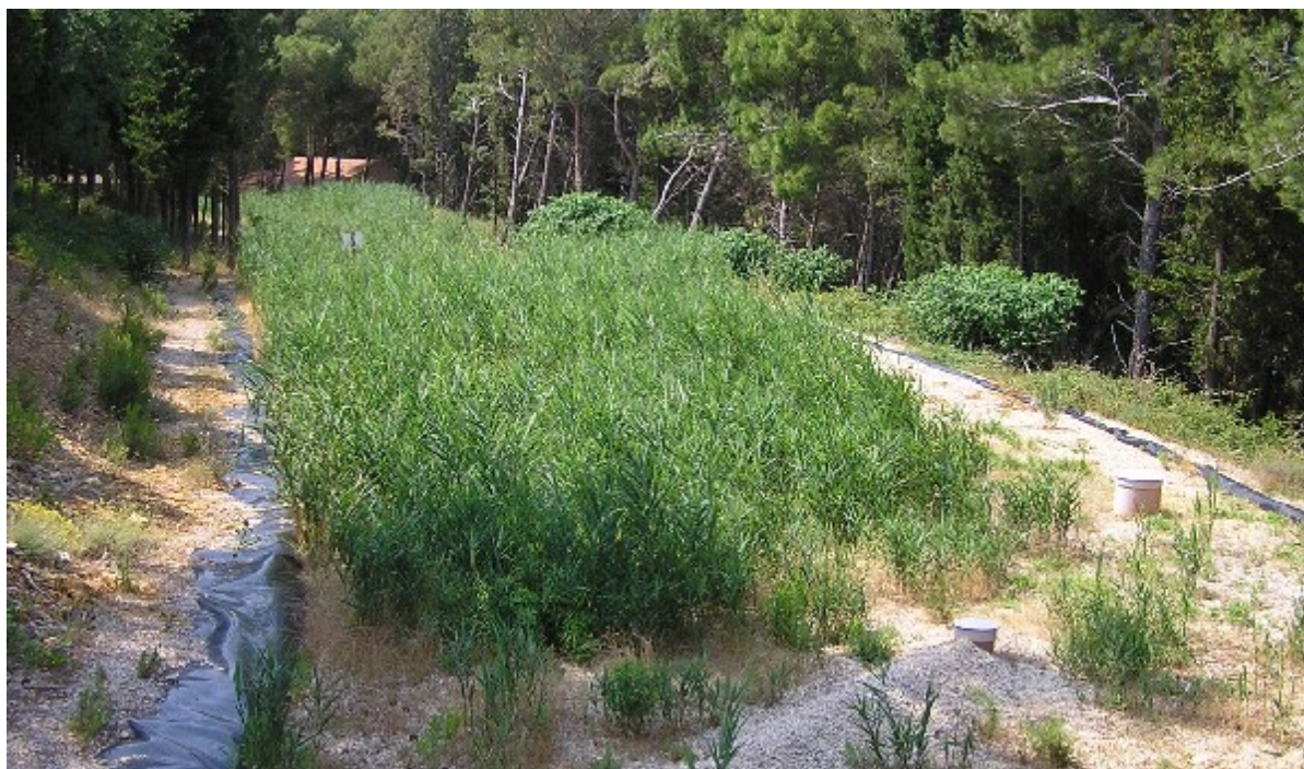
Fig. 1 Constructed wetland for treatment of wastewater of the motoring camp Bijar [11]
