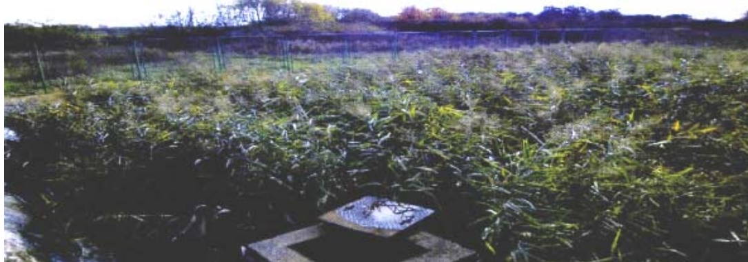
Fig. 4 Constructed wetland Vinogradci
