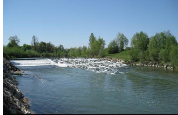
Fig. 2 Boulder ramp [7]
