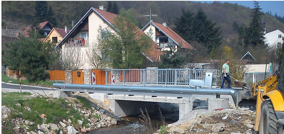
Fig. 4. Reconstructed bridge in the village Píla (May 2013)
