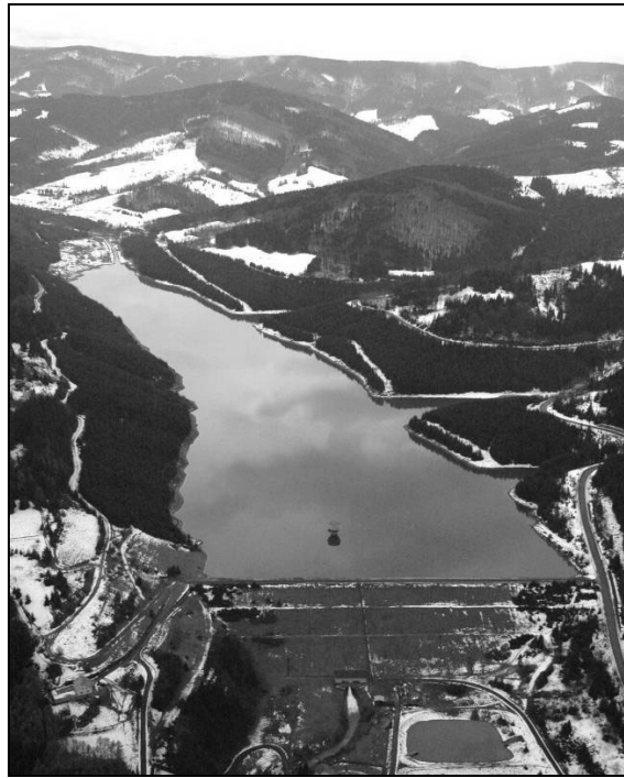
Fig. 6. View of the Karolinka Dam and Reservoir
