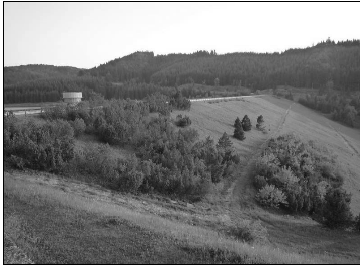
Fig. 15. View of the downstream face of Karolinka embankment Dam
