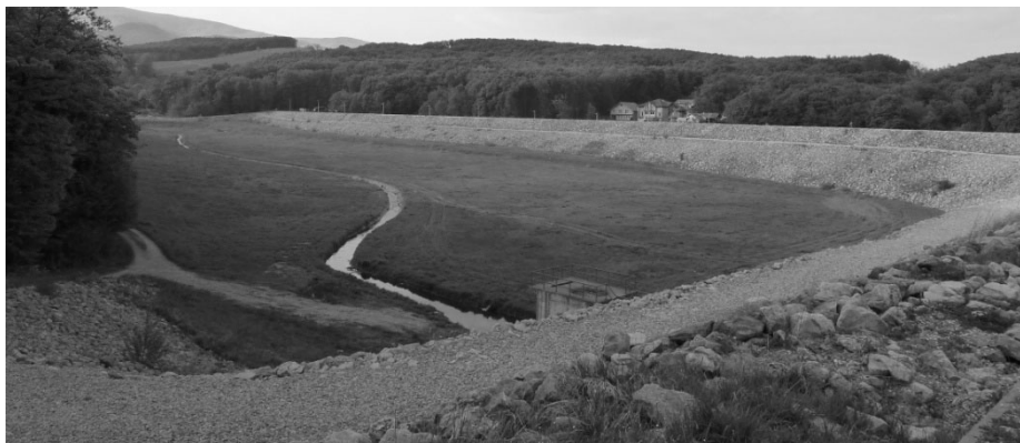
Fig. 2. Jazbina Dam and retention basin
