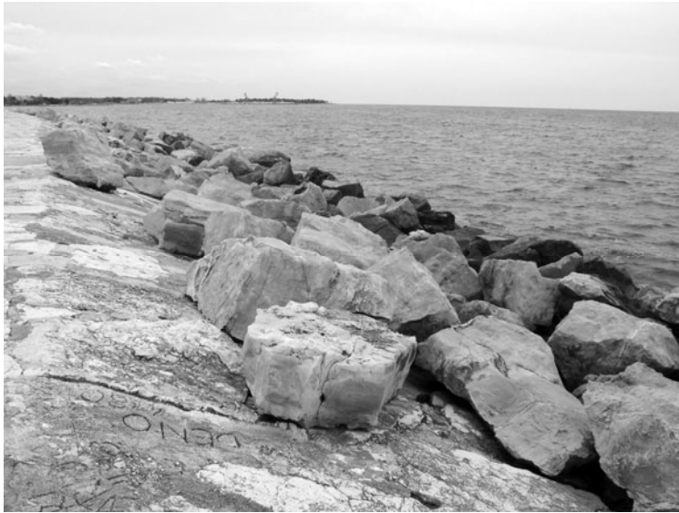
Fig. 5. A view to the slope of the primary breakwater in Umag
