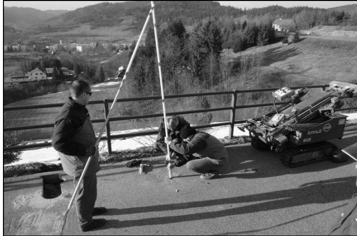
Fig. 8. Installing of probe of the EIS method into sealing core dam
