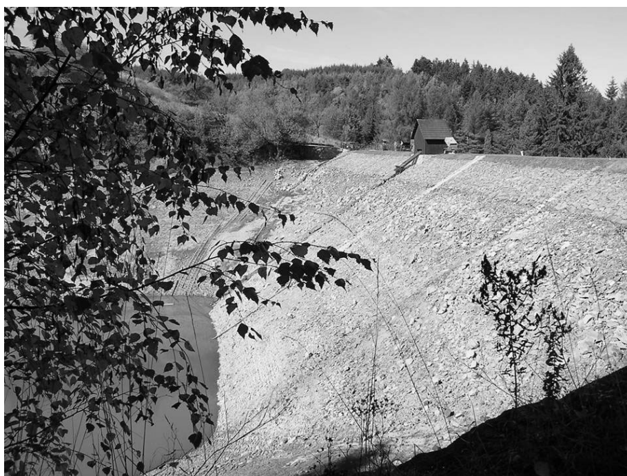
Fig. 8. Dam Rozgrund during reconstruction of bottom outlet (Photo: Bednárová E.)
