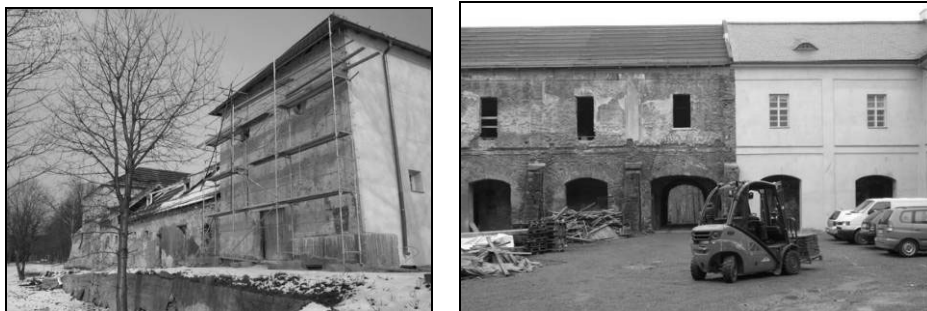
Fig. 9. Rychvald Castle under reconstruction
