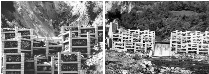
Fig. 14. Screw chack-dam (barrage) type Herheulidze (torrent Arvati and torrent Pena)
