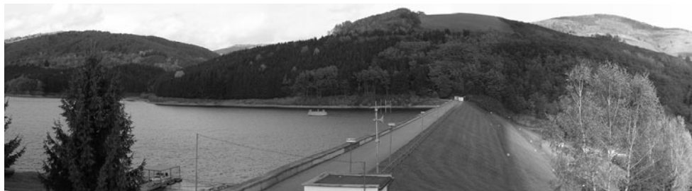
Fig. 4. Dam Klenovec (Photo: Panenka P.)
