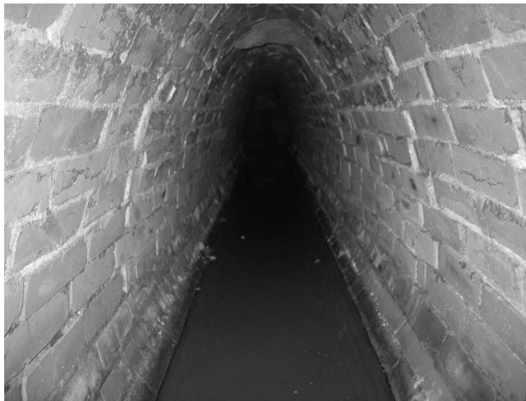
Fig. 2. Brick intercepting sewer in Hallera Street in Gdańsk
