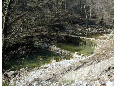
Fig. 8. Consolidation steps (barriers)
