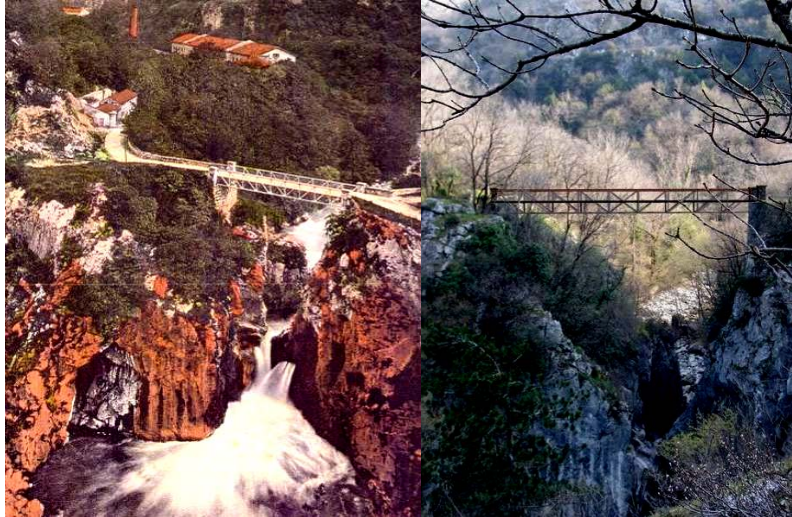
Fig. 13. The bridge leading to the Žakalj Mill: once and today
