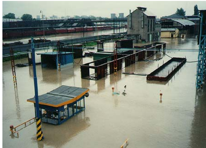
Fig. 1. Flooded railway station “Ostrava hlavní nádraží” in 1997 by Odra River
