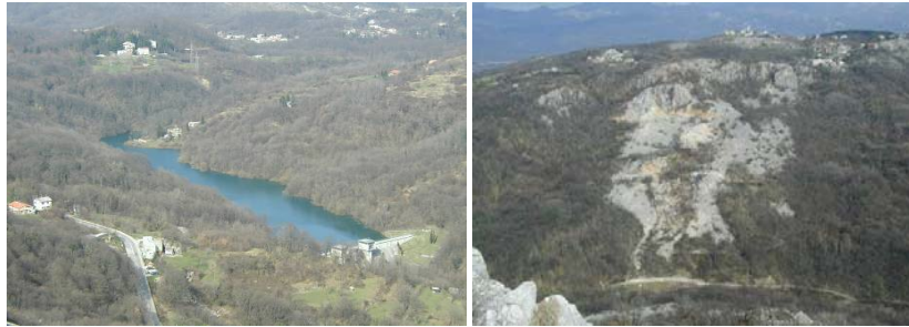
Fig. 4. Valiči reservoir with the concrete dam Fig. 5. Grohovo landslide
