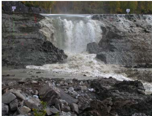
Fig. 1. Formation of an opening in an embankment dam as a consequence of overtopping [3]
