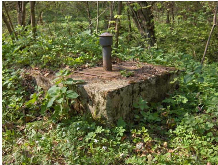
Fig.1. Typical water intake of a rural waterworks (Hum na Sutli, 2008.)
