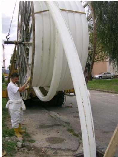
Fig.2. Reparation of the sewer system Stupava DN300 by Compact Pipe
