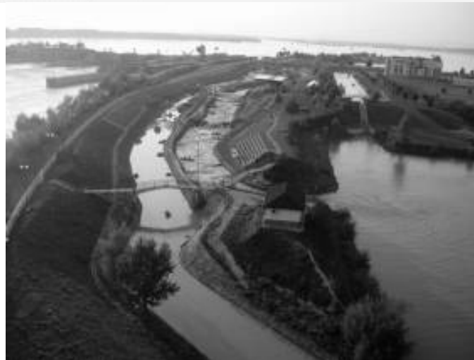
Fig. 3. Water sports complex in Čunovo
