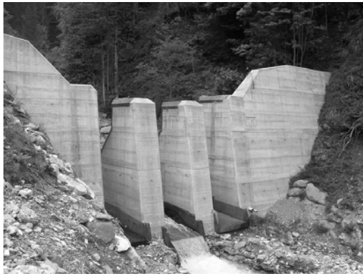
Fig. 1. Example of debris flow barrier made of structural concrete (view upstream)
