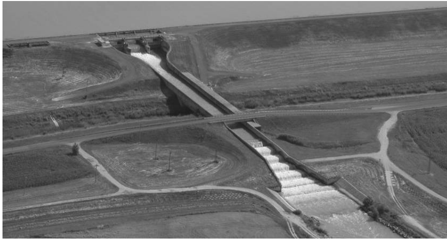
Fig. 1. The Dobrohošť intake structure
