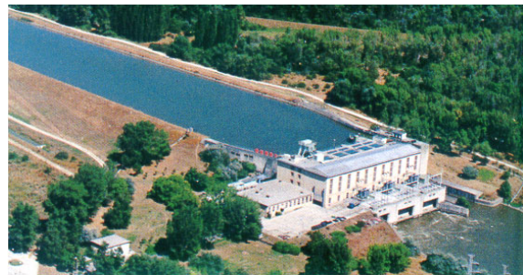
Fig. 3 The hydropower plant Madunice
