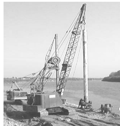
Figure 2 Construction of geotechnical diaphragms and piles
