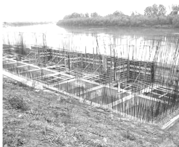
Figure 4 Front wall reinforcement (end of September 2003)
