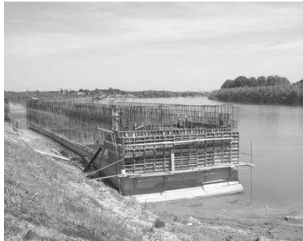
Figure 11 Reinforcement of walls (May 2004)
