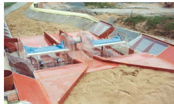
Little water power plant Gries, Salzach River M_I = 20
