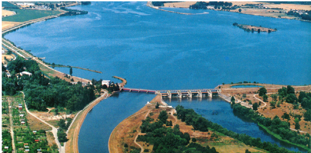
Fig. 2 Intake structure of HPP Madunice intake channel and weir Drahovce
