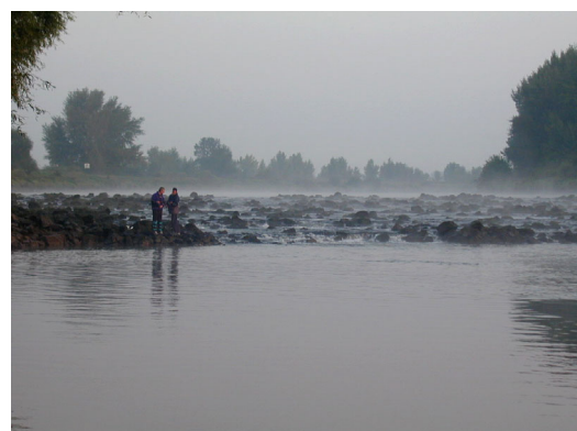
Fig. 5 The chute at the end of the HPP Madunice outlet channel (downstr.view)
