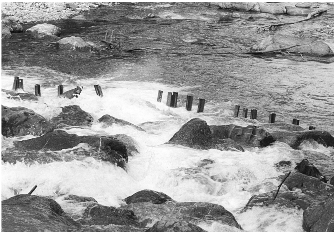
Figure 2 Example of a fish migration barrier due to bed erosion downstream of a ramp
