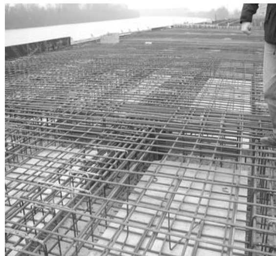
Figure 13 Reinforcement of upper slab (December 2004)
