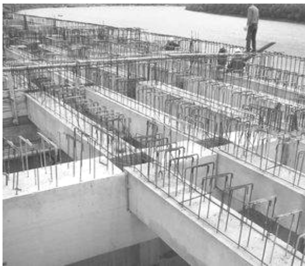
Figure 12 Girders of upper grid (September 2004)
