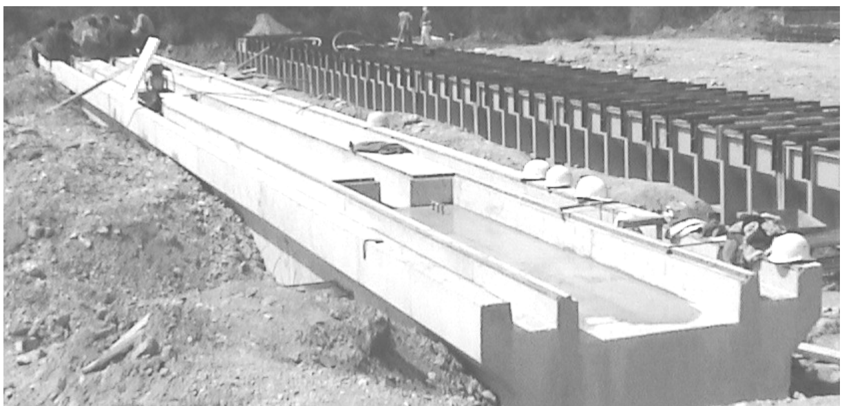
Figure 4 One horizontal girder completed and the other under construction
