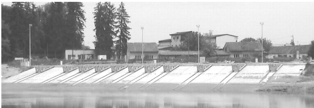
Figure 7 The constructed slipway structure with trolleys
