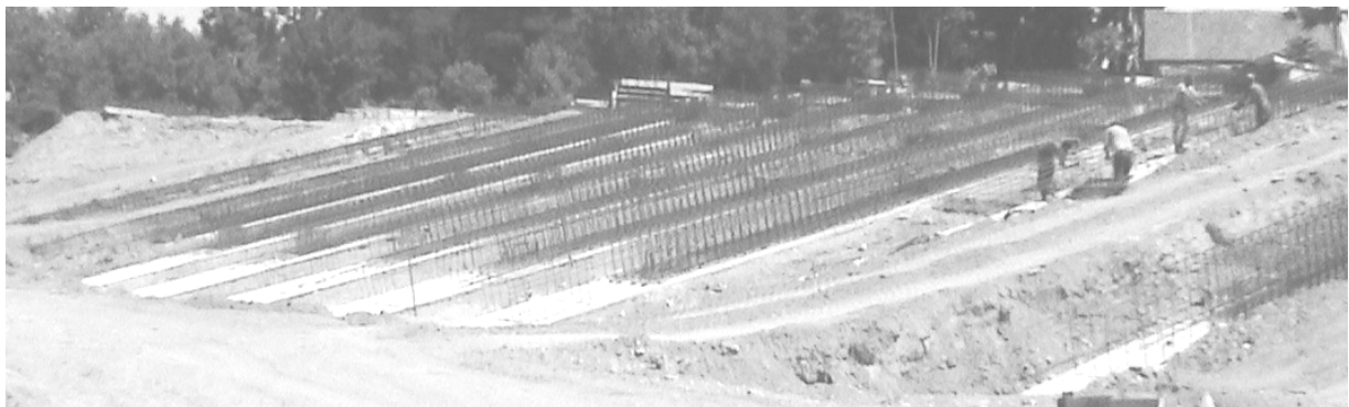
Figure 3 Inclined part of the slipway structure under construction
