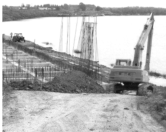
Figure 3 Front wall reinforcement (beginning of September 2003)
