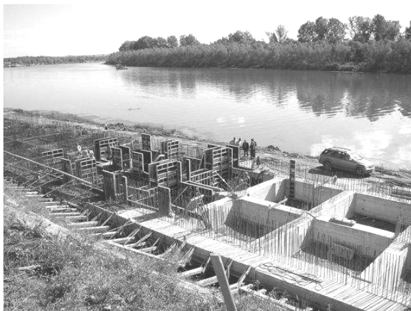
Figure 8 Construction of cross walls (September 2003)
