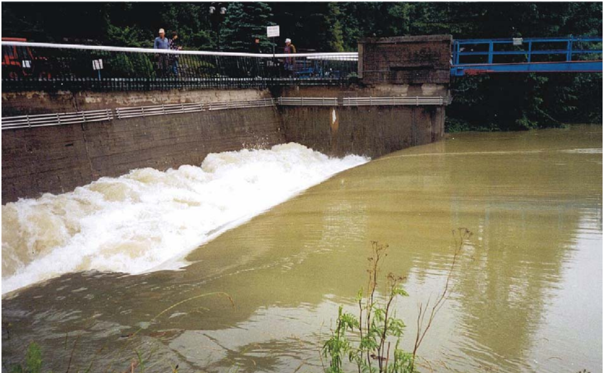
Fig. 1 Spillway outflow about 110 \text{ m}^3/\text{s} on July 9, 1997 (Odra River Board Agency archive)
