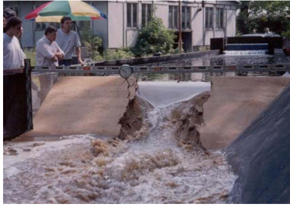
Fig. 5a Breach from the downstream - time 120 s
