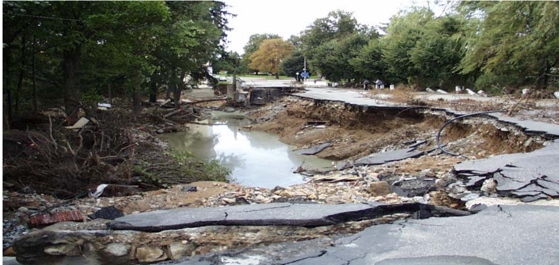
Fig. 5 Damage of asphalt dam crest of Lany dam after its overtopping for 8 hours
