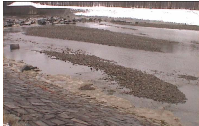
Fig. 4: Watercourse section with the pear-shaped structure – a physical model; a problematic watercourse section due to silting under the weir in Vyšné Lhoty.
