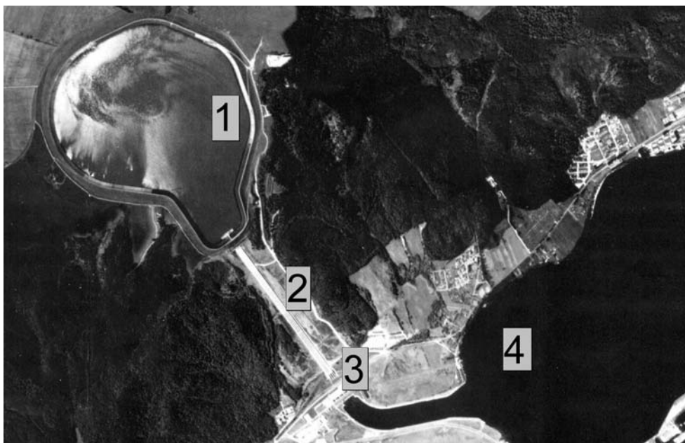
Fig. 1. Aerial view on the pumped storage power plant Żarnowiec (1-upper reservoir, 2- pipelines, 3-power plant building, 4-Żarnowieckie Lake).
