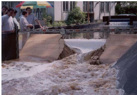
Fig. 6a Breach from the downstream - time 140 s
